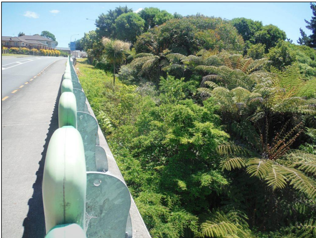
Plate 4 View of the stream crossing at the Paremuka Stream showing tree ferns and weedy area adjacent to the bridge
