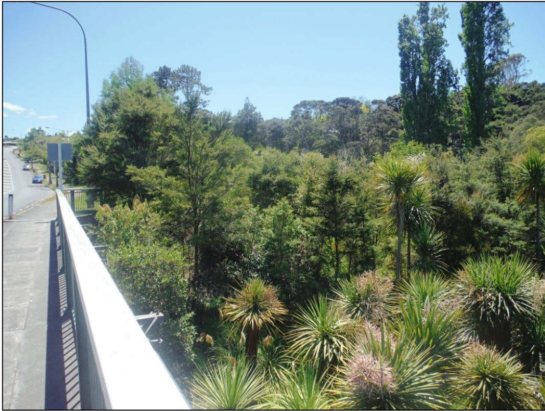
Plate 3 View of proposed stream crossing at the Opanuku Stream showing young planted natives
